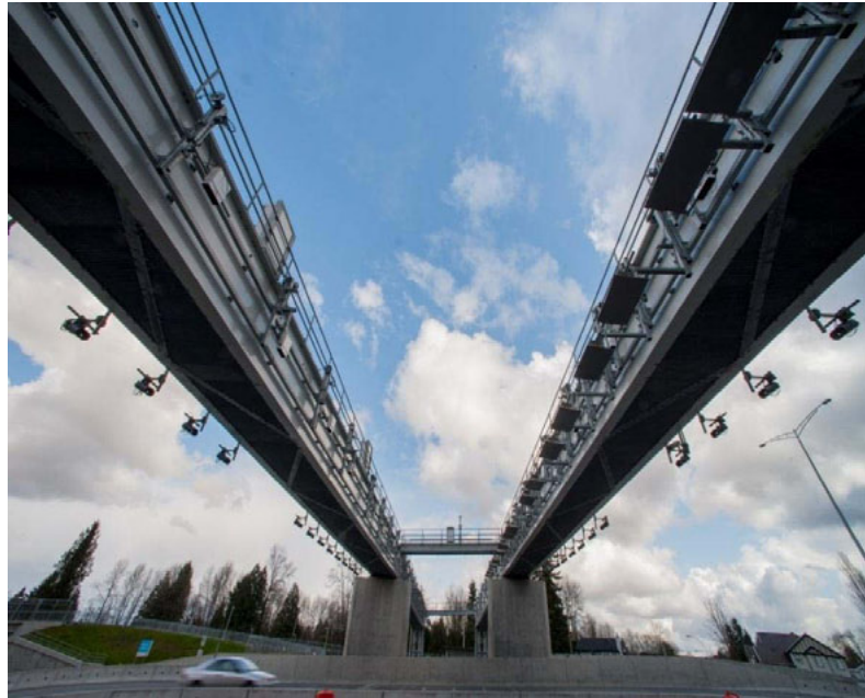
The toll gantry located on the east side of the Port Mann Bridge in Surrey spans 75 metres across Highway 1.
