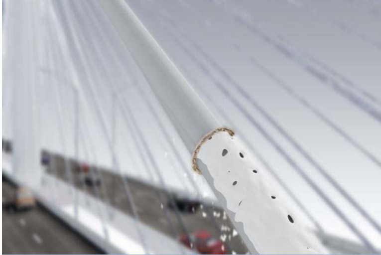
Cable collars, a snow and ice control measure, are installed on the Port Mann Bridge and keep traffic flowing smoothly during a series of heavy winter storms during 2013/2014.
