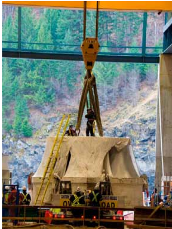
One of the two turbine runners being installed at the Waneta Expansion Project
