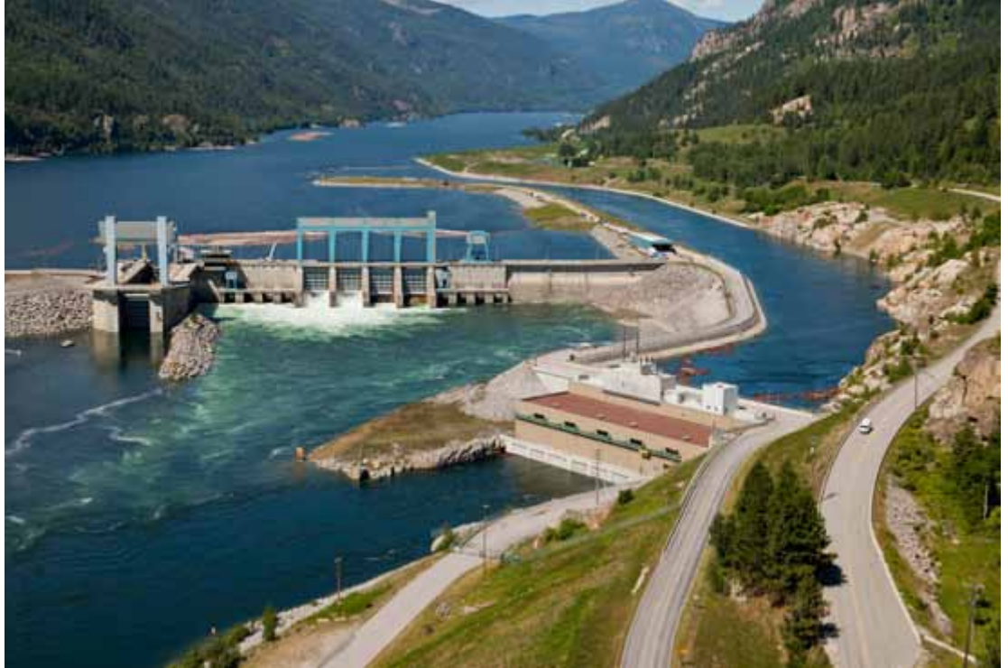
Arrow Lakes Generating Station with BC Hydro's Keenleyside dam in the background
