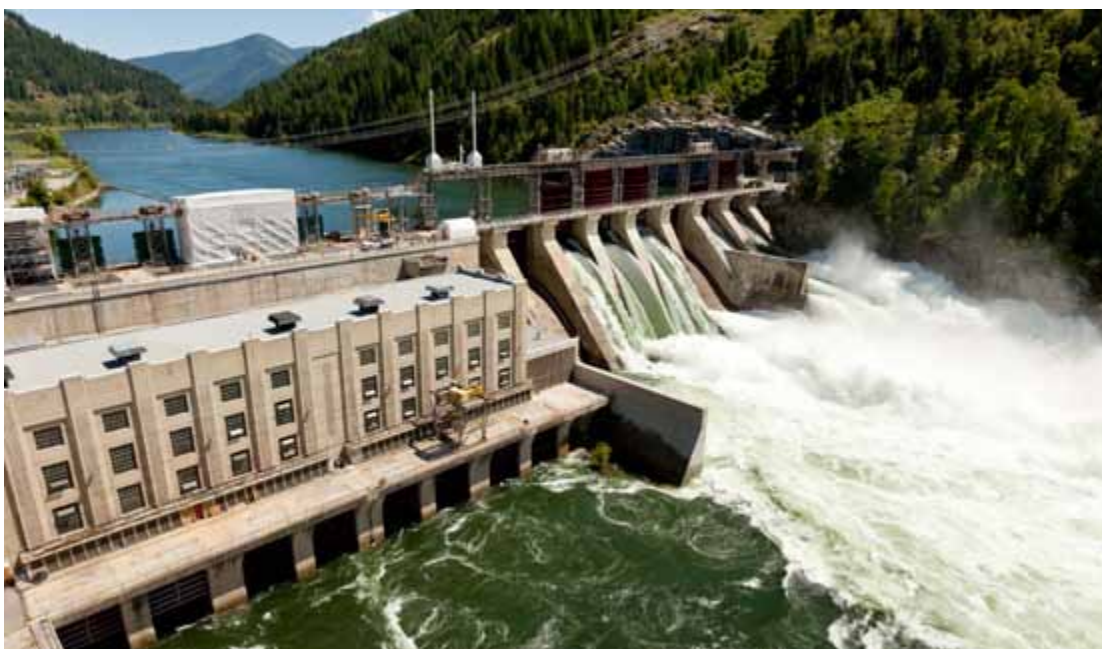
Brilliant Dam and Generating Station
