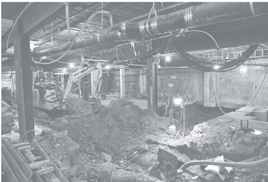
Renovations at the Marble Arch will make the building more energy efficient.
