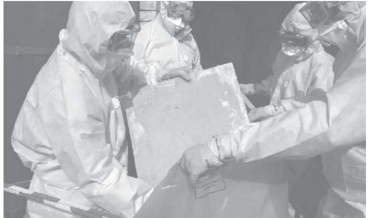
The Asbestos Management Toolkit assists non-profit housing providers in creating their own asbestos management program.
