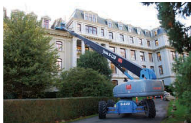
Repairs at St. Ann's Academy
