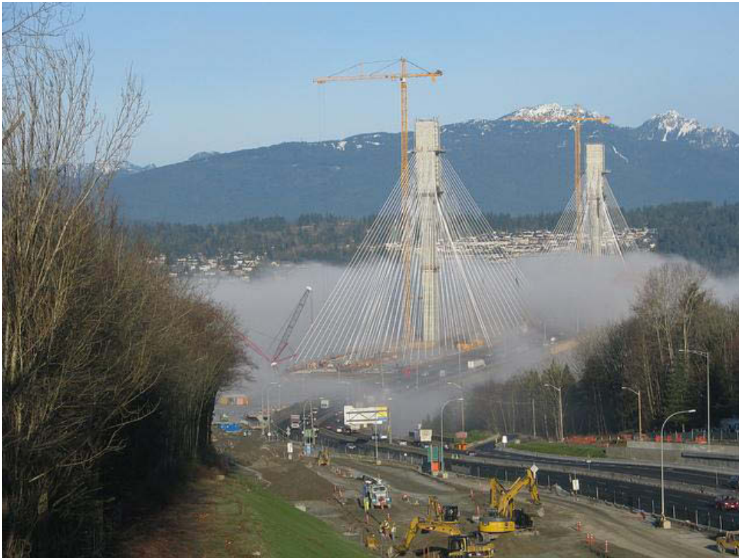
The new Port Mann Bridge rises from the fog with construction work along the approaches to the crossing seen in the foreground.
