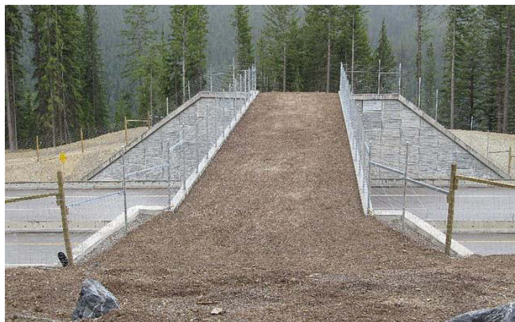
This wildlife overpass is located 17 kilometres east of Golden on the Trans-Canada Highway and will improve safety in the area by helping to prevent vehicle collisions with local wildlife.
