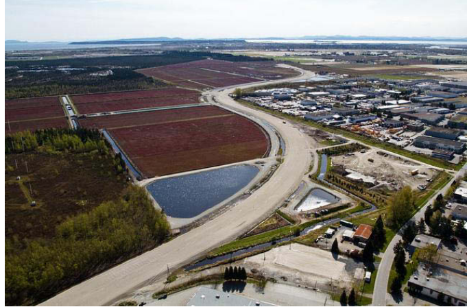
This image shows preliminary road base construction along the SFPR looking southwest towards Deltaport.
