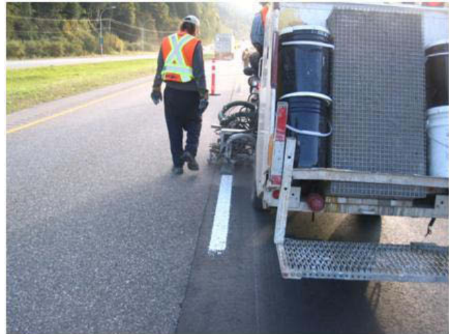
Enhanced reflectors and line markings are installed along sections of Highway 1 between Langley and Hope.
