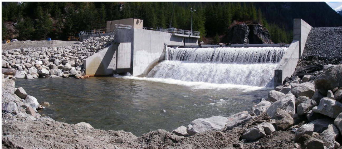
The intake for the award-winning East Toba hydro project, constructed by an Independent Power Producer in partnership with the Klahoose First Nation. The facility delivers 715,000 megawatt hours per year of clean power.
