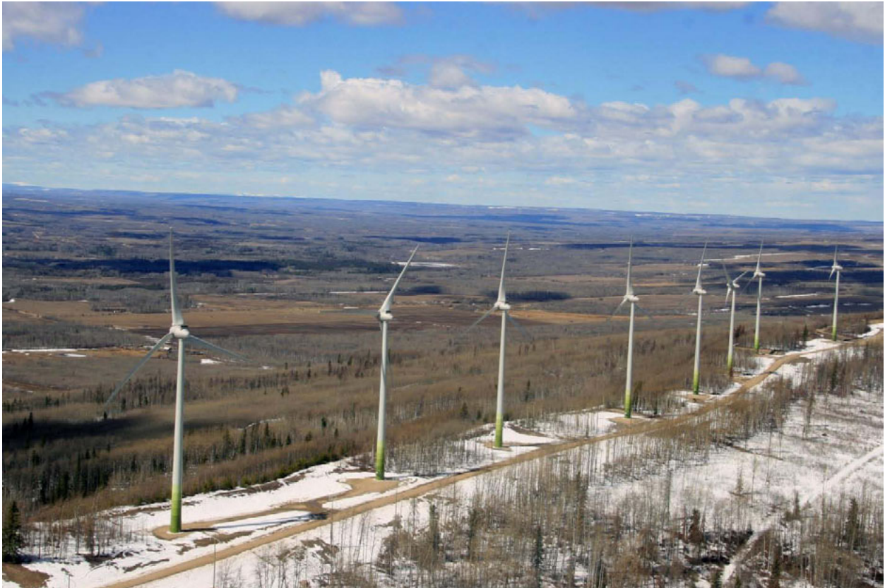
The 102 megawatt Bear Mountain Wind Park, near Dawson Creek, which includes 34 windmill towers, has been operational since 2009.
