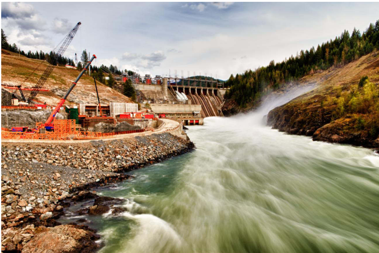
Construction continues on the Waneta expansion project, a partnership between Columbia Power Corporation, Fortis Inc. and the Columbia Basin Trust. The new facility is expected to be operational by the spring of 2015.
