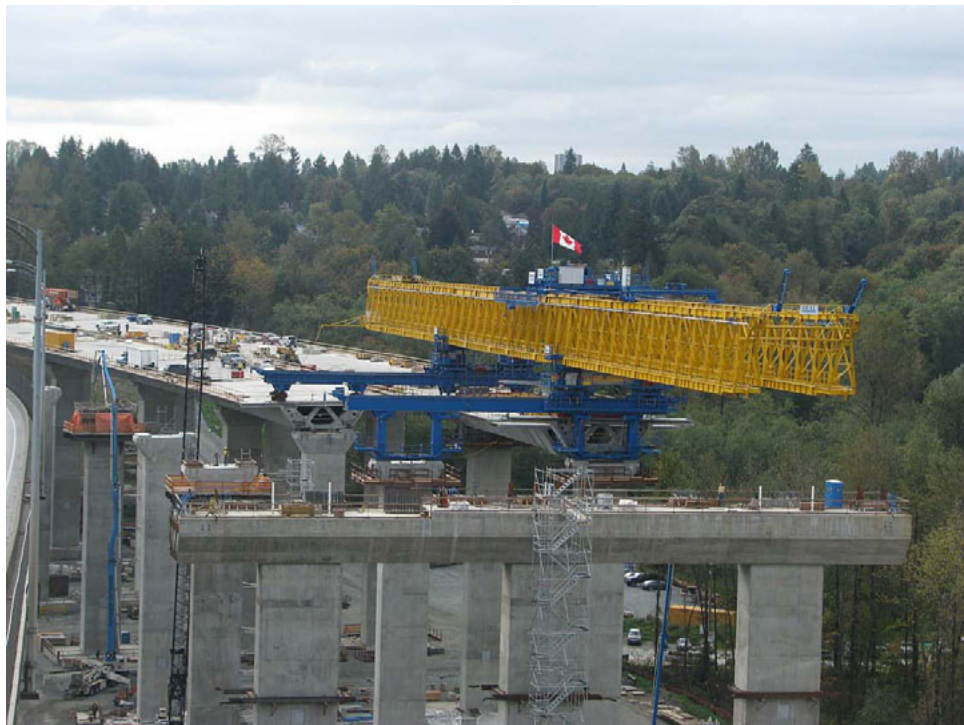
Positioned on the south approach of the new Port Mann Bridge the 720 tonne gantry lifts 90 tonne pre-made sections of the bridge deck with a hoist and moves them horizontally into place.
