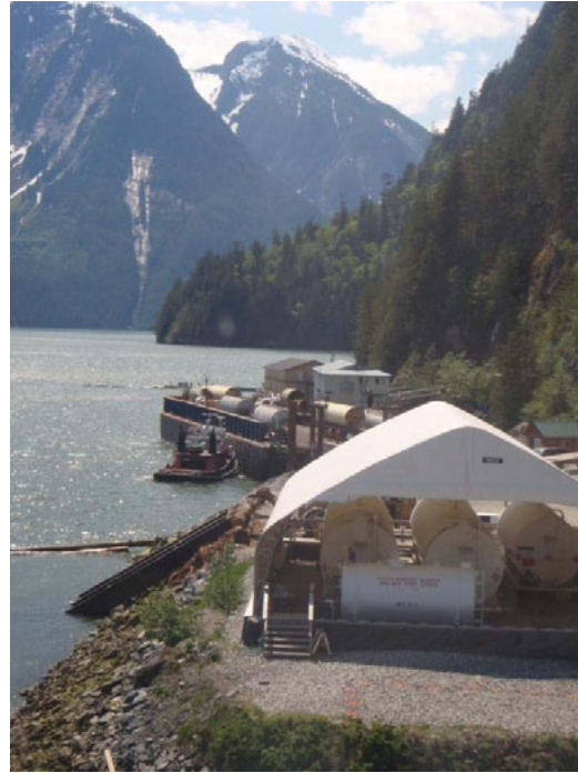
Barge landing at the East Toba River Montrose Creek Hydroelectric Project near Powell River
