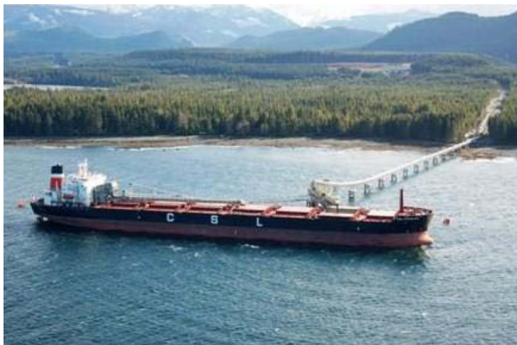
The CSL Acadian at the Orca Sand and Gravel Quarry Marine Terminal near Port McNeill, Vancouver Island
