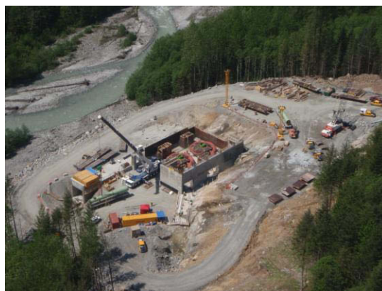
Construction of the East Toba River Montrose Creek Hydroelectric facility north of Powell River
