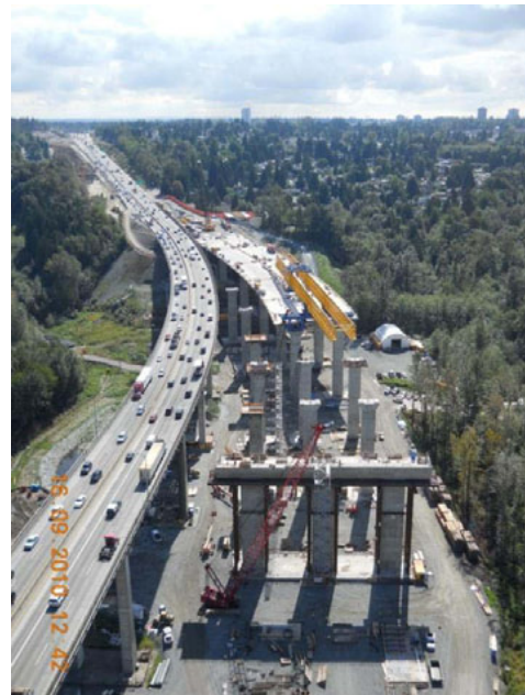
Construction of the Port Mann Bridge-Highway 1 Project in the lower mainland
