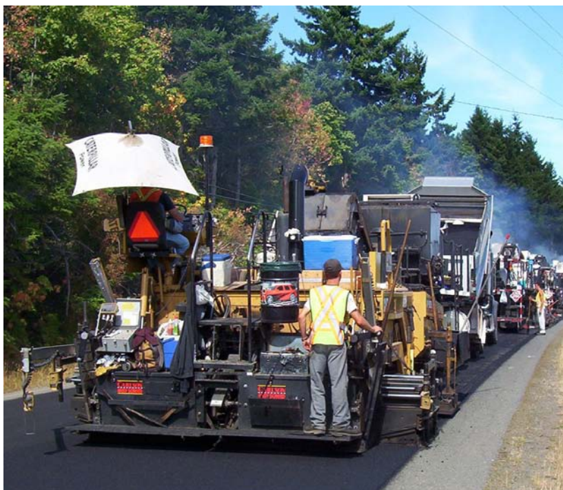
Hot-in-place recycling revitalizes highways and saves taxpayers' money.
