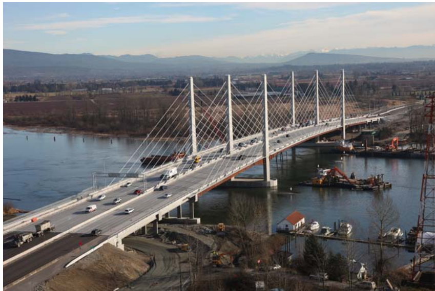
The new Pitt River Bridge is cable-stayed, which minimizes the number of piers in the water to protect the marine environment.
