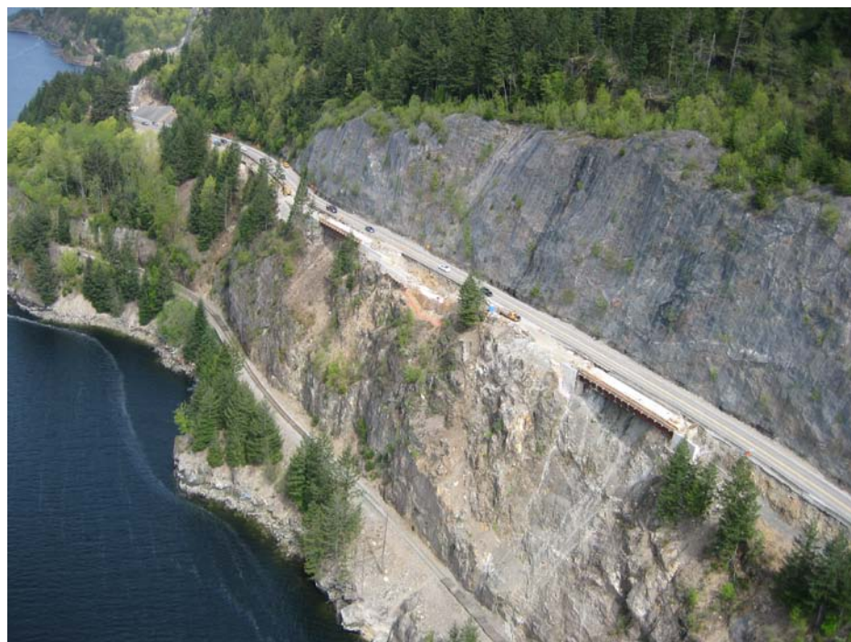
The Sea-to-Sky Highway Improvement Project used half-bridges and retaining walls as an alternative widening strategy to rock slope excavation, which would have resulted in unacceptable delays to the travelling public during construction.
