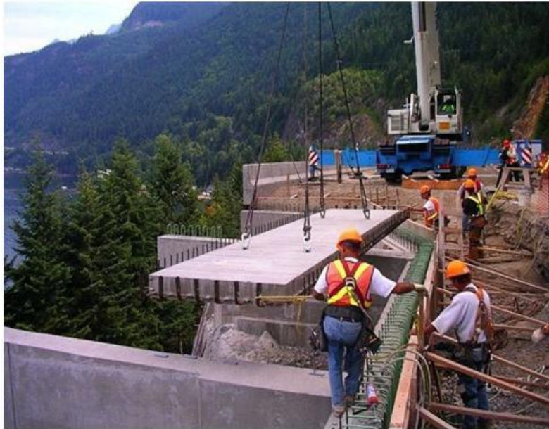
Construction on the Sea-to-Sky Highway Improvement Project
