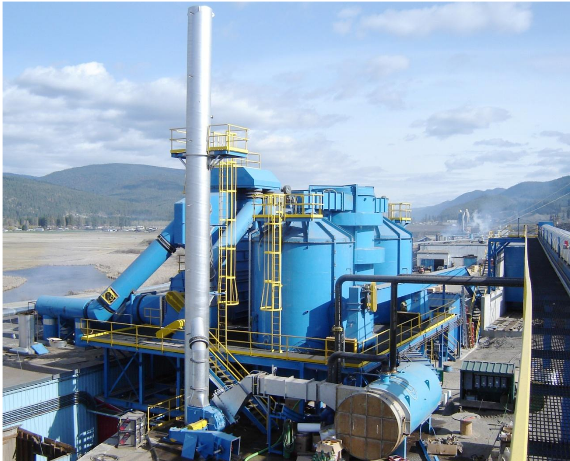
Nexterra Gasification Plant at Hefley Creek near Kamloops, B.C.
