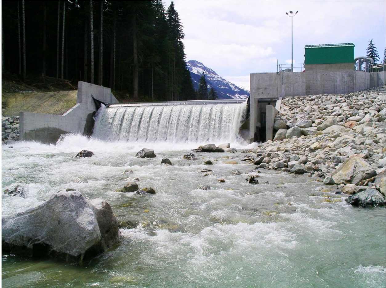
Innergex run-of- river hydroelectric dam and powerhouse on Rutherford Creek, B.C.
