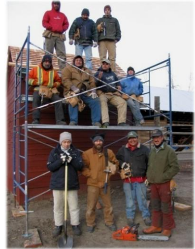
Displaced resource workers carry out repairs and upgrades at provincial historic sites under a JOP-funded project.
