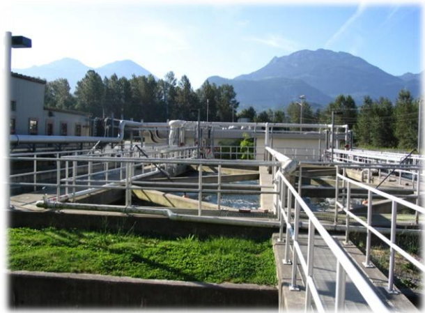
The Ministry funds the construction of water treatment plants, like this one in Port Edward, all around the province.
