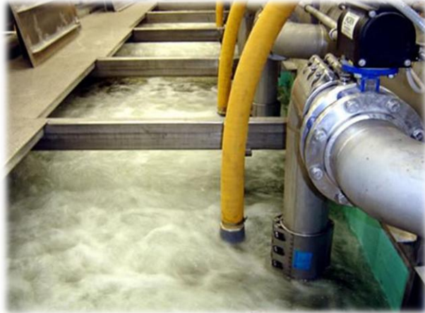
A water treatment facility in Kamloops provides clean drinking water for the city's residents.
