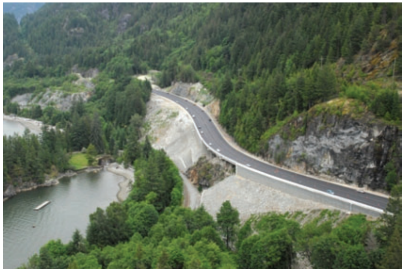
Sea-to-Sky Highway Improvement Project – showing the use of mechanically stabilized earth walls and ‘half bridges’ to widen highway just south of Porteau Cove Provincial Park.
