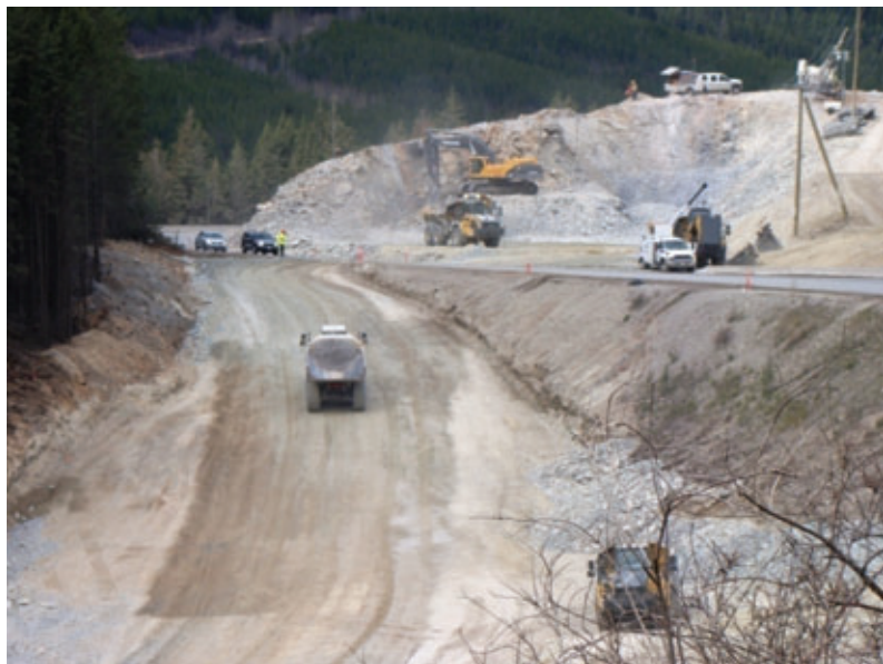
Removing large rock cut east of Mt Hunter Bridge.
