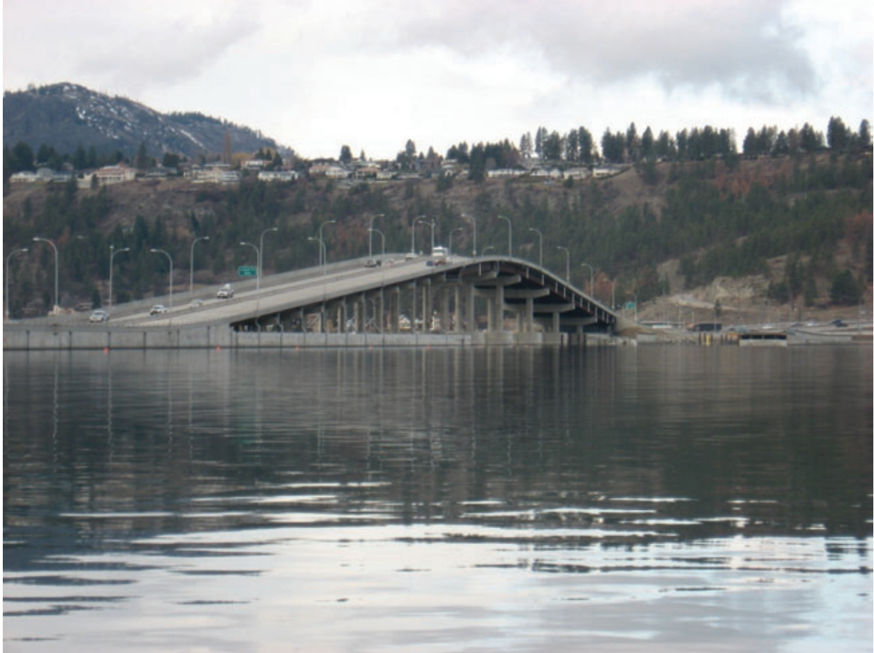
View of the William R. Bennett Bridge taken from City Park, on the east side of Okanagan Lake.
