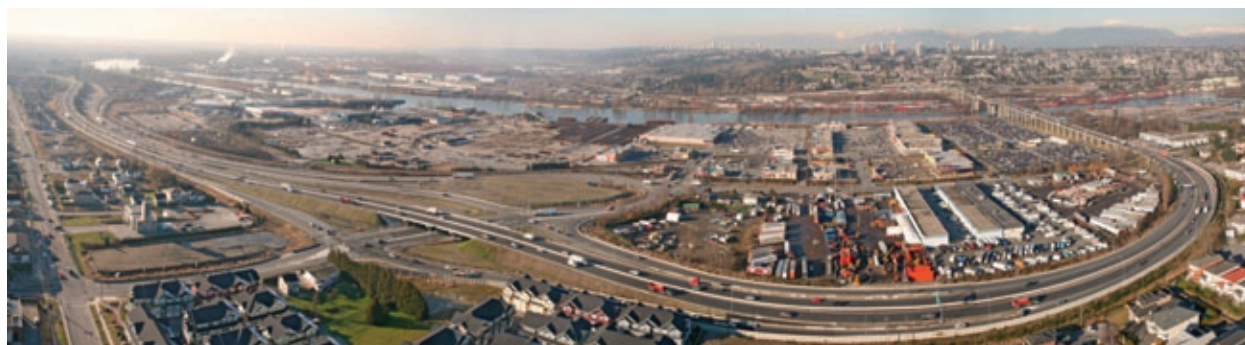
Border Crossing Program - New completed interchange at Highway 91A and Howes Street in New Westminster.
