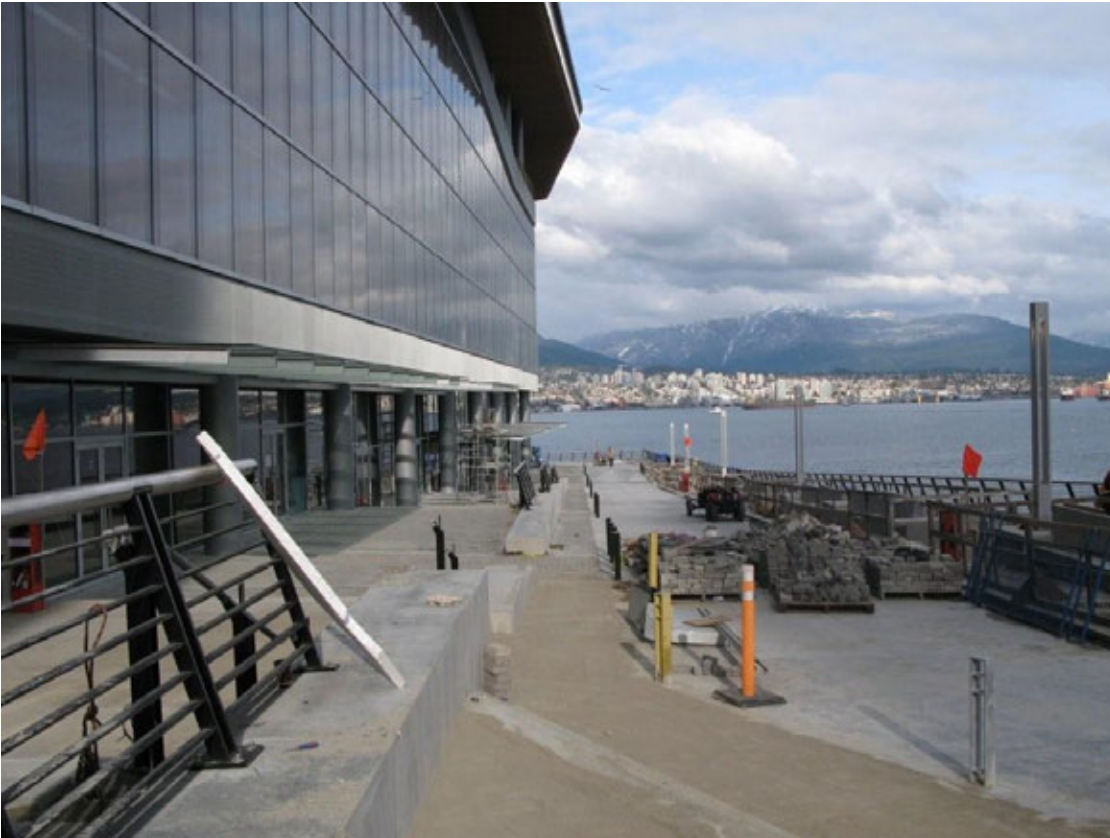
Vancouver Convention Centre construction
