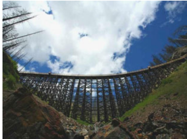
A rebuilt trestle in Myra Bellevue Provincial Park
