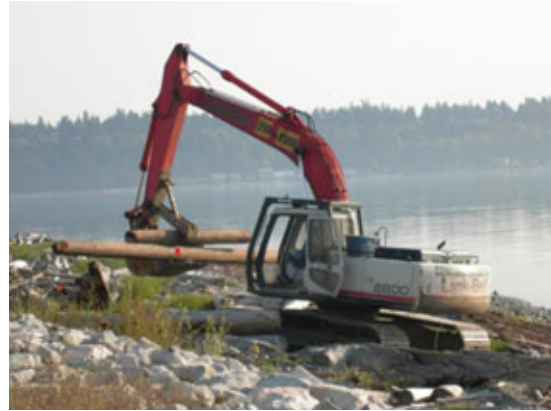
An excavator cleans up creosote-contaminated logs in Boundary Bay Wildlife Management Area, Delta/Surrey
