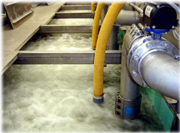
A water treatment facility in Kamloops providing clean water for the city's residents.
