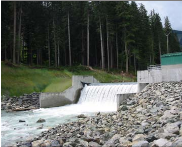
Run of river hydro power generation at Rutherford Creek, B.C.
