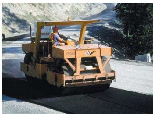
A compaction roller compacting freshly laid asphalt.
