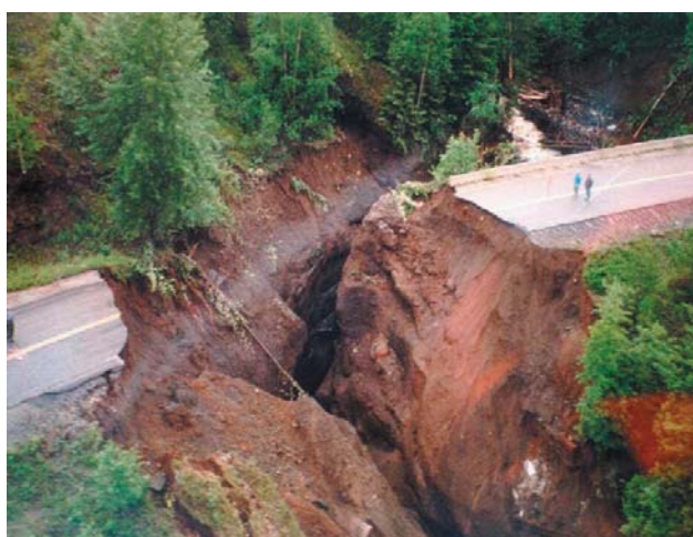
Flood and slide damage
