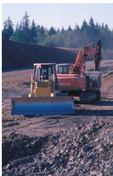
Road construction near Cumberland
