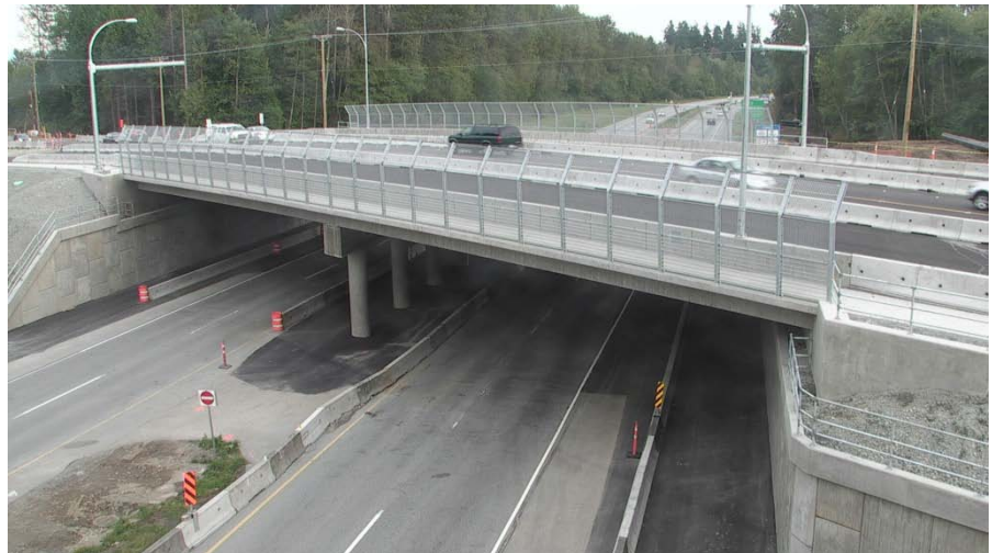
Photograph showing the new interchange at Highway 99 and 16th Avenue in Surrey.
