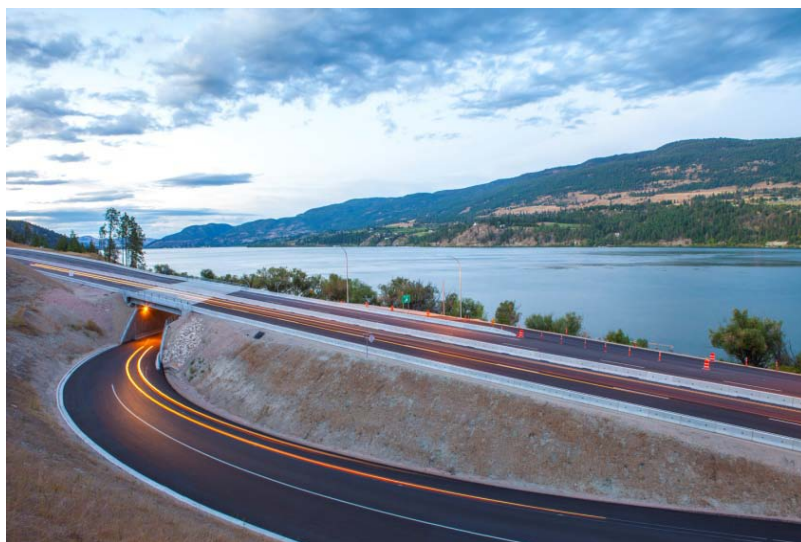
A time lapse photograph shows the new Wood Lake Overpass and the on-ramp to the Pelmeash Parkway passing underneath. The Overpass and Parkway were part of improvement work undertaken along the heavily-used section of Highway 97 between Winfield and Oyama.
