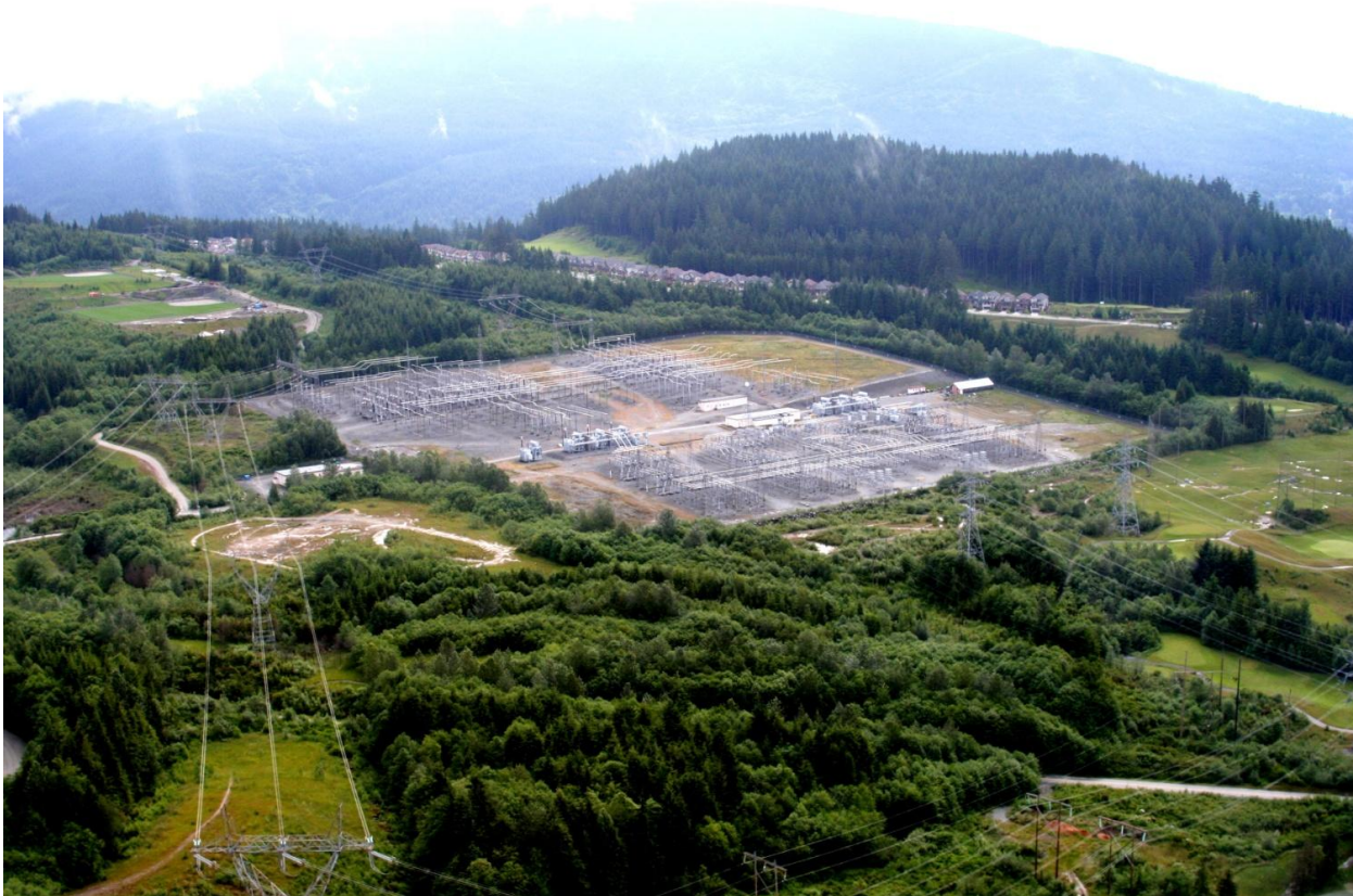
The Meridian substation at Westwood Plateau in Coquitlam is being upgraded as part of the new Interior to Lower Mainland 500kV transmission line. By allowing for more efficient transmission of electricity from Merritt to the Lower Mainland area, when it is finished in 2015 the 247 km line will save enough energy to power approximately 80,000 homes.
