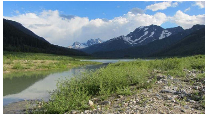
Coursier Lake Dam decommissioning compliance inspection site
