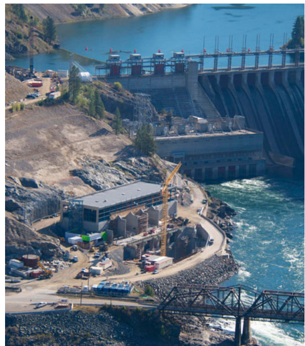
Aerial view of the new Waneta Expansion Project powerhouse
