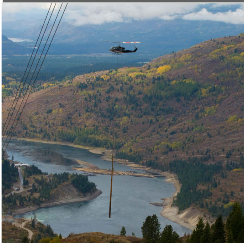
A helicopter placing poles for the new Waneta Expansion 230kV transmission line
