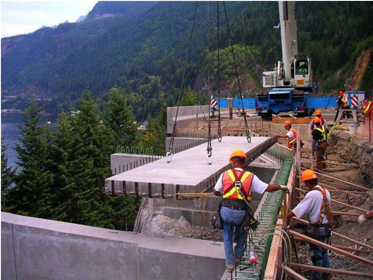
Construction on the Sea-to-Sky Highway Improvement Project in the Lower Mainland
