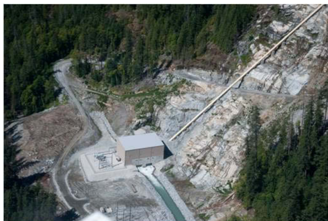
East Toba Montrose hydroelectric facility taken during a compliance inspection in August 2011.
