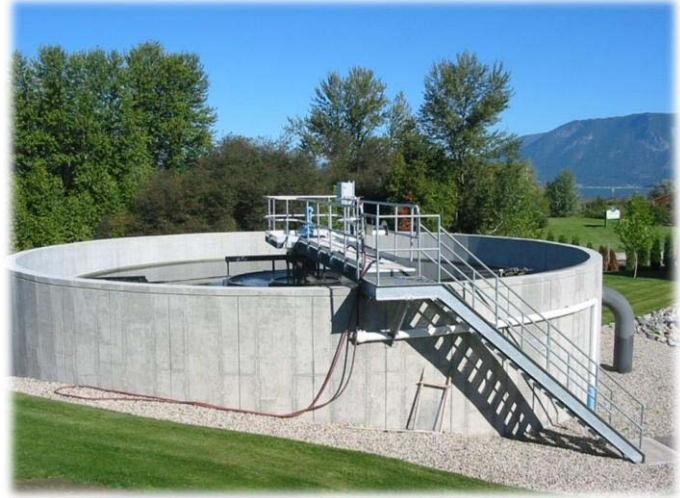
A Ministry-funded water treatment plant in Salmon Arm, B.C.
