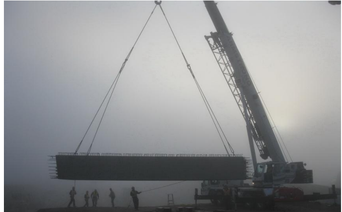
Kicking Horse Canyon Project Phase 3 West: First Girder to be erected for the Golden Donald Upper Road Underpass
