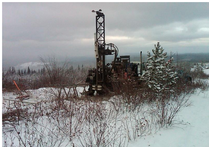
Geotechnical core sampling for the Quality Wind Project, near Tumbler Ridge
