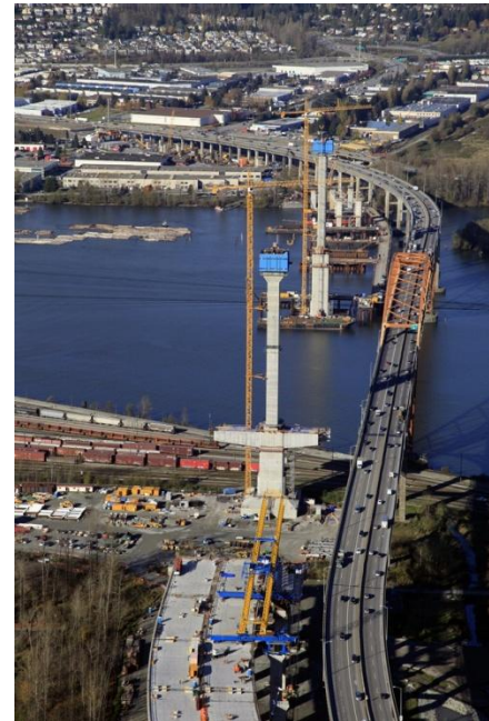
Construction of the new Port Mann Bridge as part of the Port Mann/Highway 1 Project, Lower Mainland
