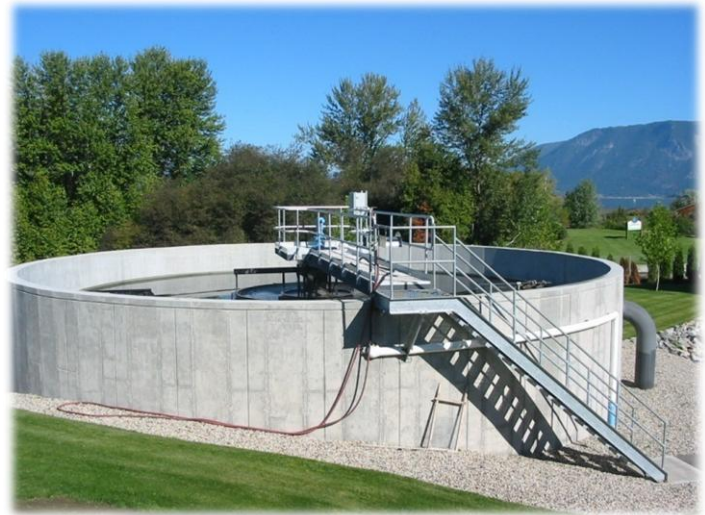
A Ministry-funded water treatment plant in Salmon Arm.
